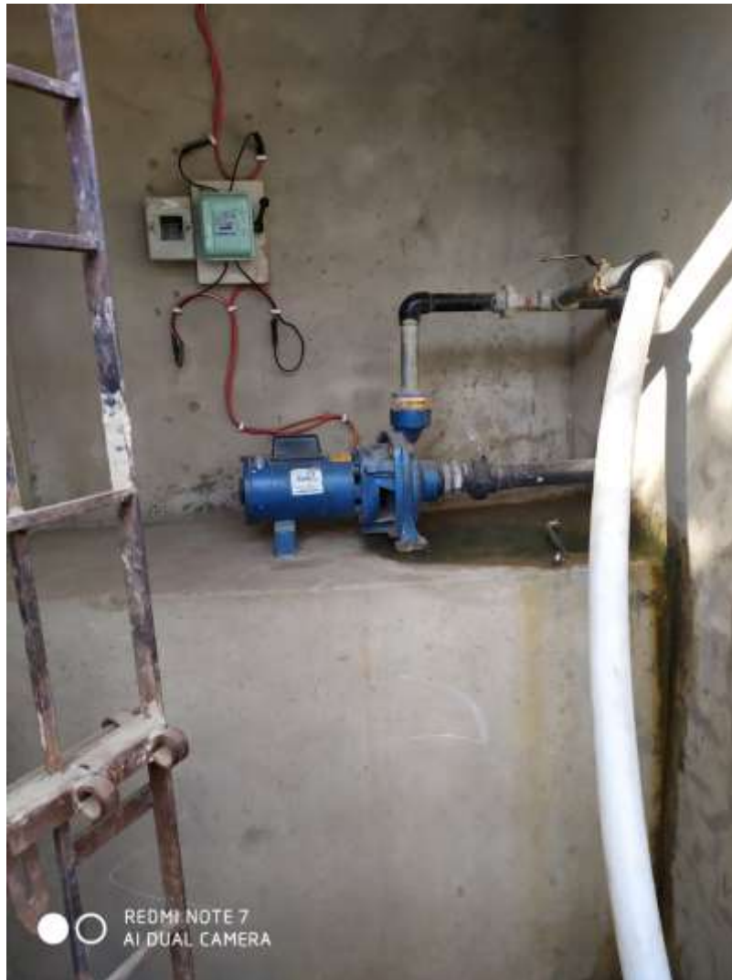
Picture 16: Solar Motor Water Pumping Machine Provided as Part of the Programme
