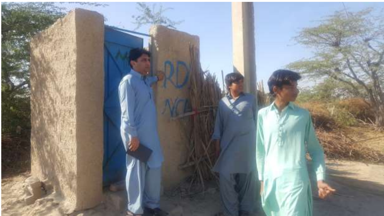
Picture 10: Latrine Supported Under the Programme
