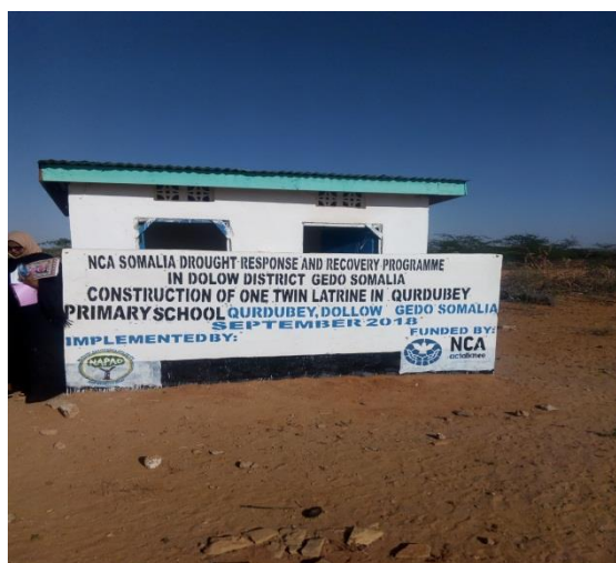
Latrines in Qurdubay Pry School
